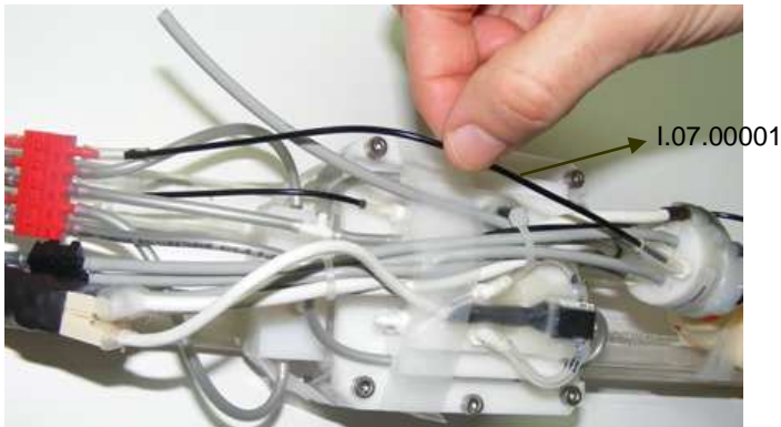
Pneumatic connection used in the other gas usage
